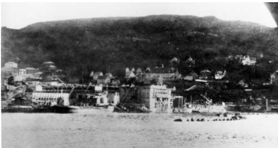
5. The U-boat shelter, looking SSE. July 1943.
