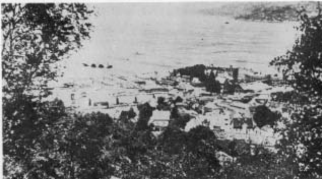
6. Nordre Vaag. German U-boat base under construction, looking north (July 1943).
